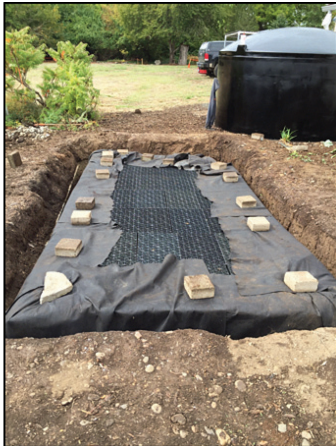
FIGURE 5. Final layer of AQUABLOX installed with pond liner and underlayment folded over the top during backfilling and compaction around the basin.
