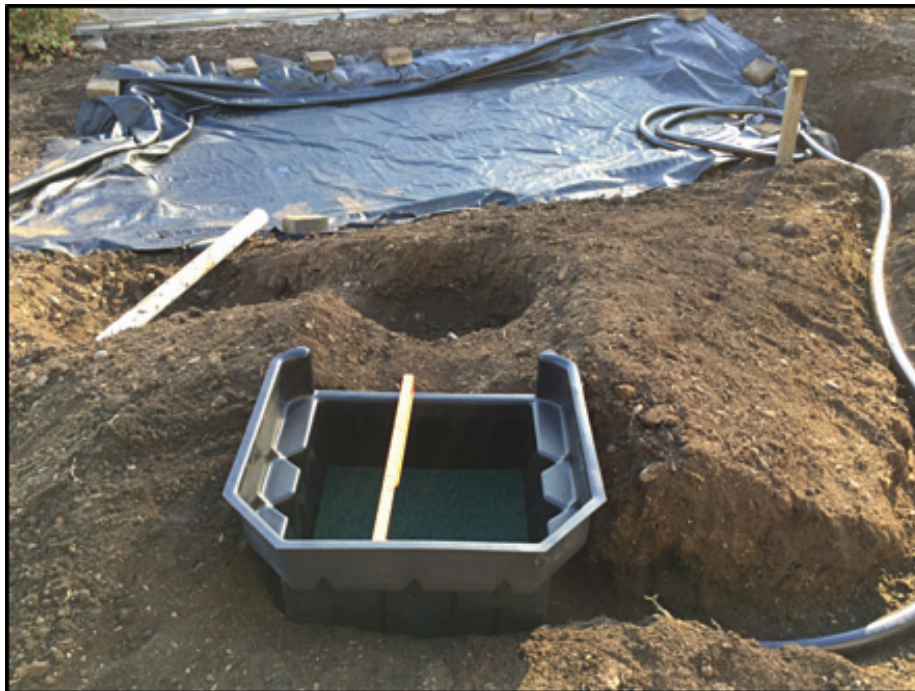
FIGURE 8. Waterfall box carefully leveled to create an even spillway at the start of the falls.
