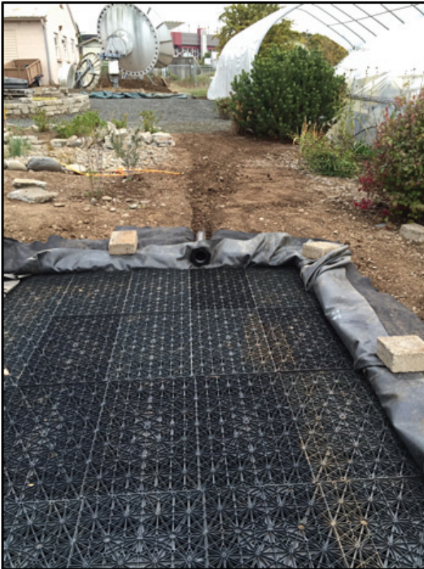
FIGURE 7. Overflow pipe fixed to pond liner at the top of the Aquablox to maximize capacity.
