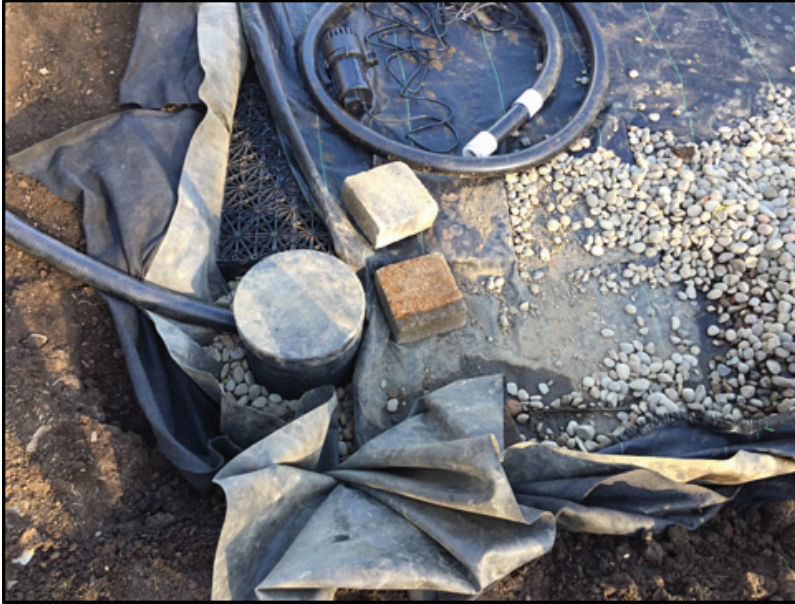
FIGURE 7. Overflow pipe fixed to pond liner at the top of the Aquablox to maximize capacity.
