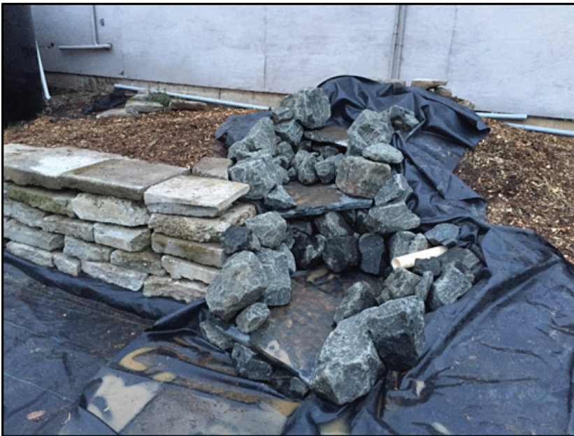
FIGURE 4. Recirculating waterfall feature built with gutter-diversion piping entering the system between the second and third spillway.
