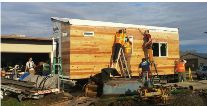
FIGURE 3: Traditional construction techniques were used including a vapor barrier, flashing, and wood siding.
