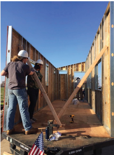
FIGURE 2: Students supporting the walls and securing them in place.
