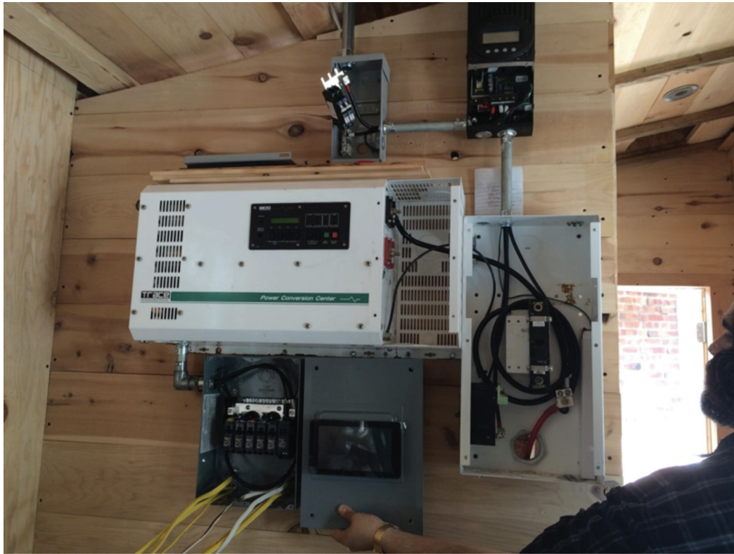
FIGURE 13: Installation of main solar PV electrical components.
