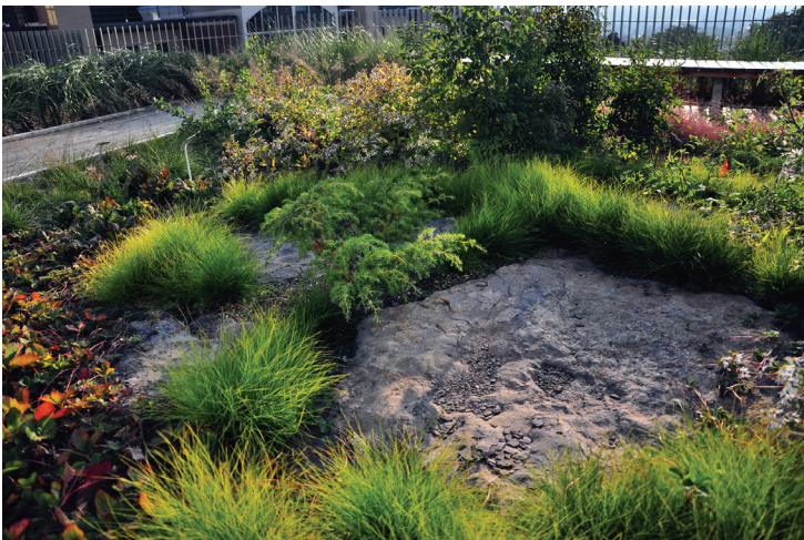
FIGURE 13: Natural stone on the green roof mimics the alvar grassland reference community's shallow bedrock, even once the plants mature. (Photo: Andropogon)
