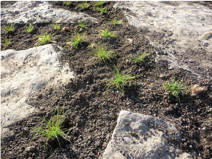
FIGURE 12: Plant spacing on the Gateway Center green roof ranged from 8-to-12-inches on center, depending on the species. (Photo: Andropogon)
