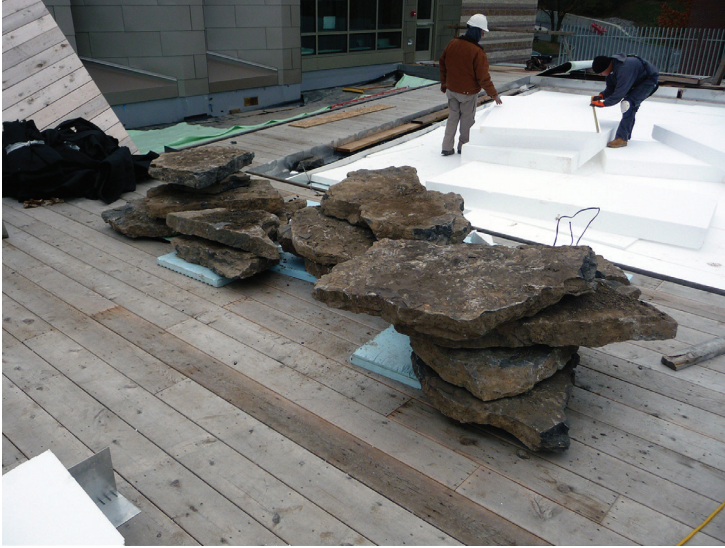
FIGURE 11: False terrain and large natural stones at the Gateway Center green roof helped create green roof microclimates, similar to conditions found in marginal reference communities. (Photo: Andropogon)
