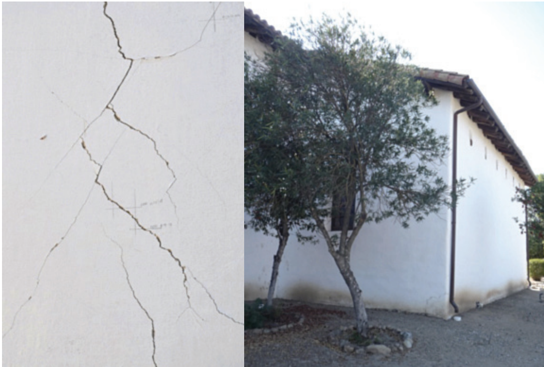
FIGURE 14 AND 15: Fig. 14 (left) – Displacement markings on east Sacristy wall, photo by author. Fig. 15 (right) – Overall view of retrofitted Sacristy looking west, photo by author.
