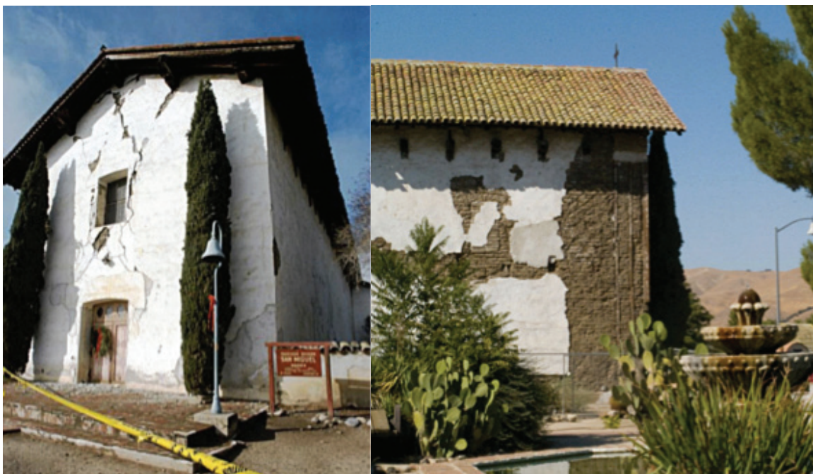
FIGURE 12 AND 13: Fig. 12 (left) – Cracks in façade immediately following 2003 San Simeon earthquake [1]. Fig. 13 (right) – View of main church during restoration, cracks repaired and plaster reapplied [1].
