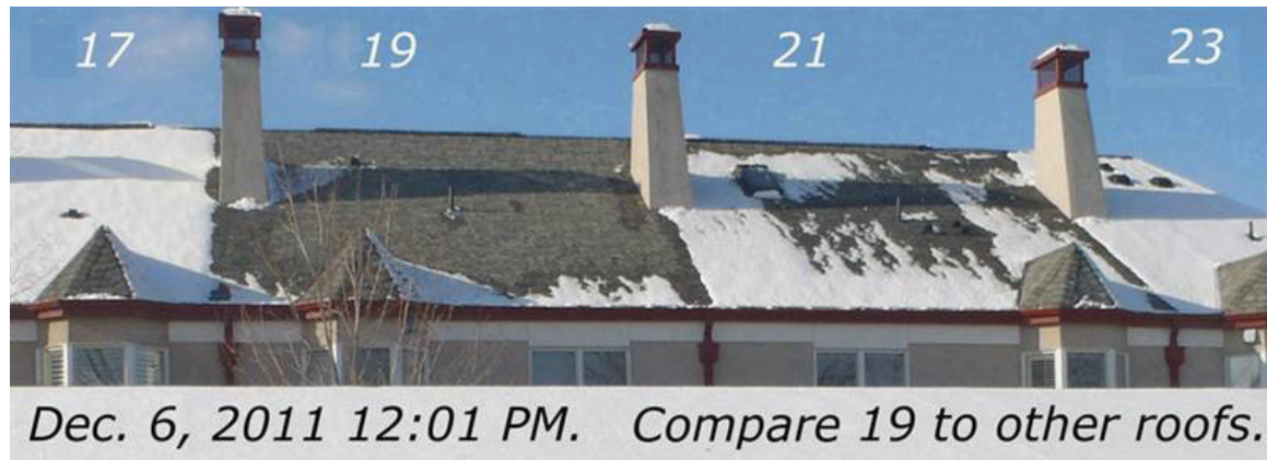
FIGURE 7: Townhouse roof snow melt patterns reveal heat loss. Reprinted from (C) HankeyandBrown.com.
