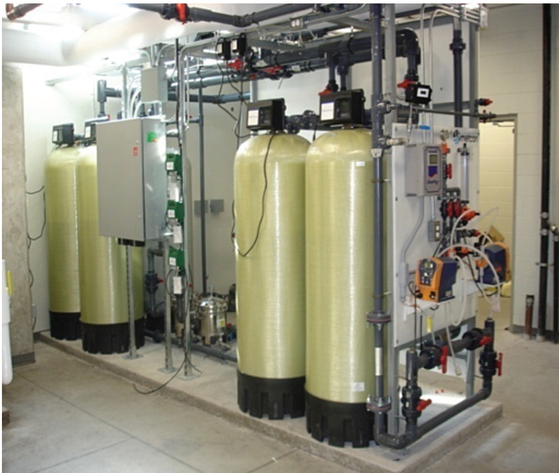
FIGURE 3. View of the filtration components (Multimedia and Activated Carbon).
