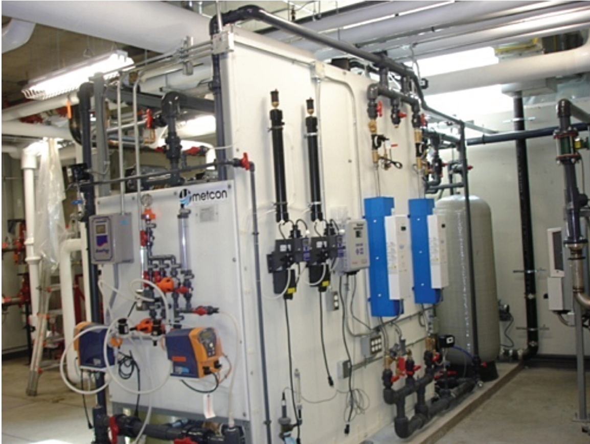
FIGURE 4. View of the disinfection components (Chlorination and Ultraviolet Light).
