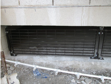
FIGURE 15: Unrestricted access for floodwaters to enter building flood storage area, Courtesy of BSC Group.
