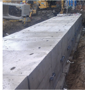
FIGURE 18: Sanitary sewer holding tank installation, Courtesy of BSC Group.
