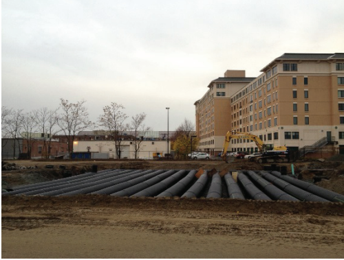
FIGURE 19: Watertight stormwater detention system, Courtesy of BSC Group.
