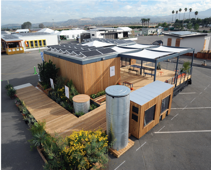
FIGURE 1: The two modules of the NexusHaus with expanding interior spaces into fully shaded outdoor decks, the aquaponics system and the thermal storage rainwater tank. (Credit: Thomas Kelsey, U.S. Department of Energy)
