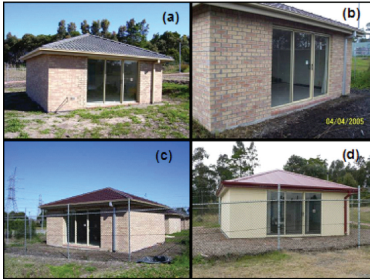
Figure 1: Housing Test Modules (with window in north wall), (a) Insulated Brick Veneer (b) Insulated Cavity Brick (c) Cavity Brick and (d) Insulated Reverse Brick Veneer.
