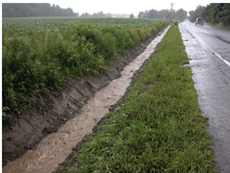
FIGURE 15: Typical road-side ditch during a rain, where water is rushing over bare clay-lined bottom, side slopes are steep, and vegetation is maintained at a low levels. Photo courtesy Cornell University, < http://climatechange.cornell.edu/re-plumbing-our-water-sheds >.
