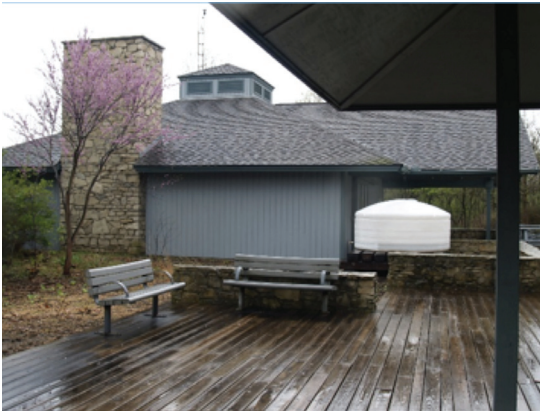
FIGURE 61: Rain Barrel collecting water off the Discovery Center roof from a spring rain. April 30, 2009. Betts 1
