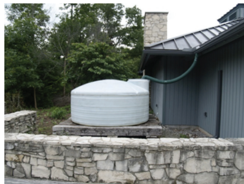
FIGURE 63: Flexible downpipe extensions are attached to the gutter and directed into the top of the rain barrel. July 10, 2015. Betts 1
