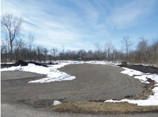
FIGURE 5: Bio-swales on March 4, 2010, indicated by the dark soil on either side of the stone lot, are visible and already retaining water from the melting snow. Betts 1
