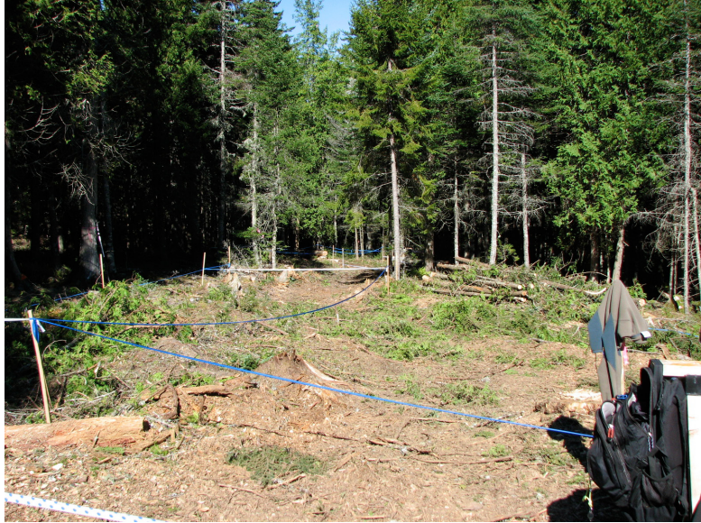
FIGURE 5: Staking out house footprint to get the solar orientation and views to the pond right.
