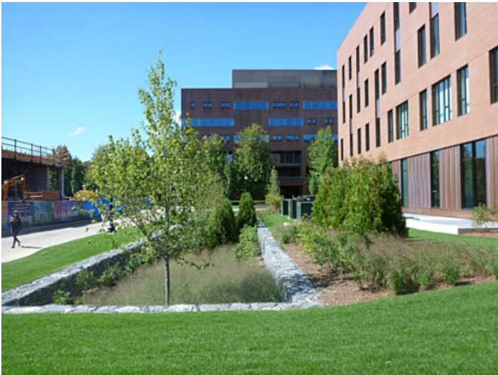
FIGURE 5: Bioretention area by Oak Hall, University of Connecticut, Storrs.
