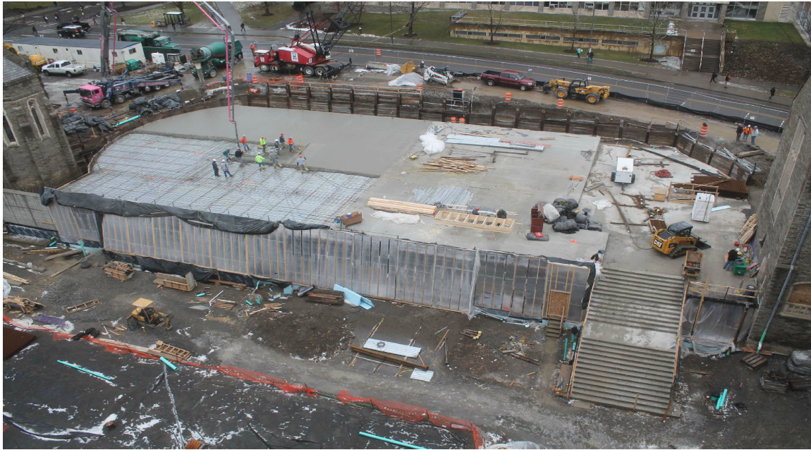
FIGURE 11: Construction of the below grade roof deck, November 2013.
