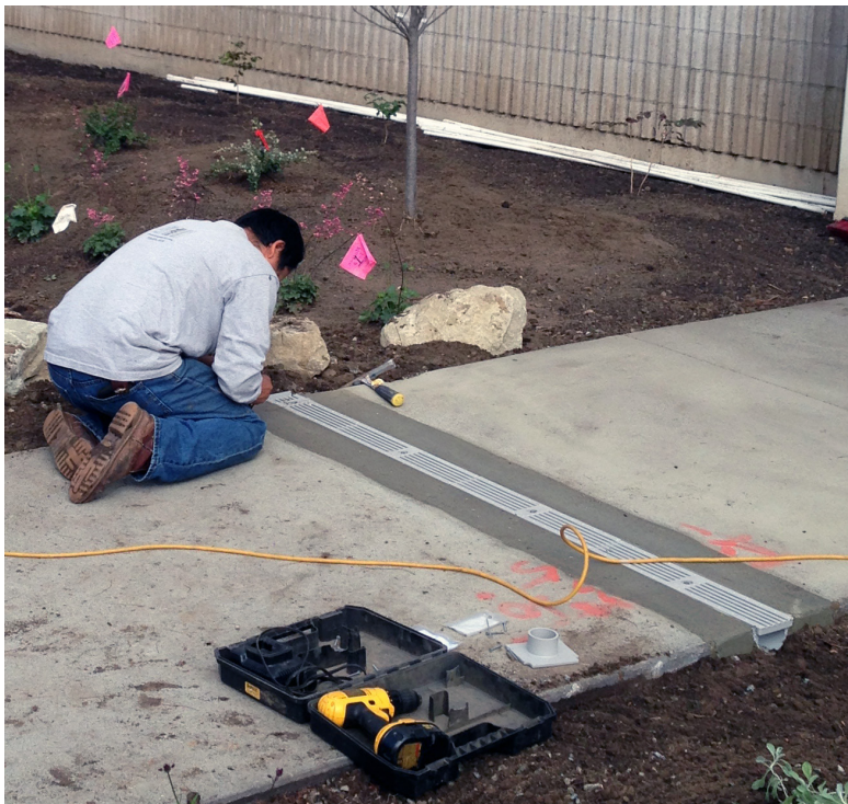
FIGURE 12. A trench drain was installed in the concrete walkway to direct surface runoff into the garden.
