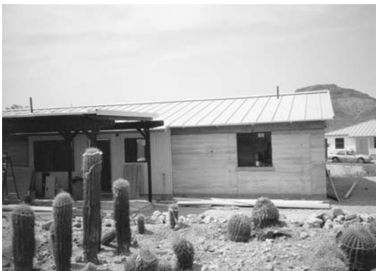
FIGURE 18. Completed rammed earth residence with roof overhangs to shade south windows.
