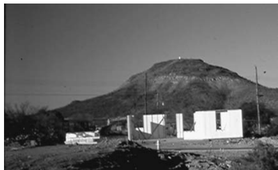
FIGURE 8. Heydon System walls under construction.
