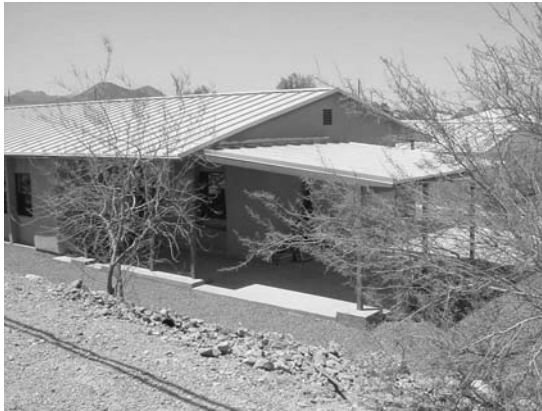
FIGURE 14. Completed straw bale residence with roof overhang to shade south windows.
