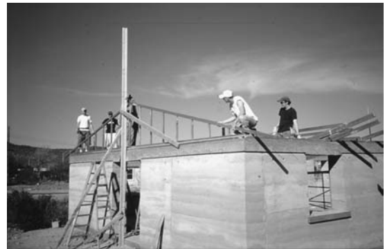
FIGURE 15. Rammed earth residence under construction.
