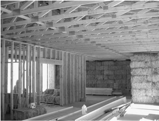
FIGURE 11. Straw bale residence under construction.
