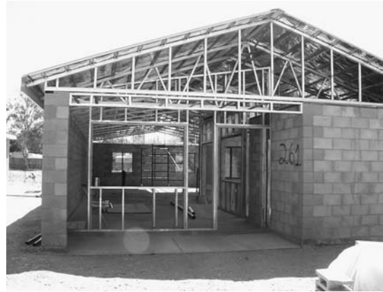
FIGURE 2. Integra Block residence under construction.
