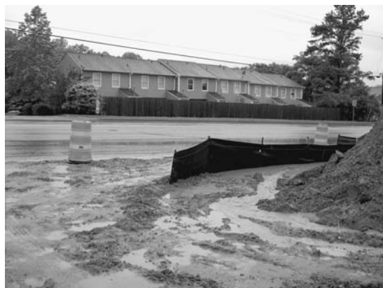
FIGURE 5. Erosion from construction sites is a major source of non-point source pollution.
