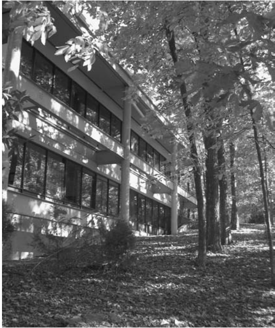
FIGURE 4. Example of a custom building designed to accommodate the topography of the site. Notice the mature trees that were preserved, approximately ten feet from the footprint of the building.
