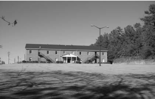
FIGURE 3. Example of a mass-graded site accommodating a building. Notice the retaining wall on the right property edge and the lack of vegetation on the site.
