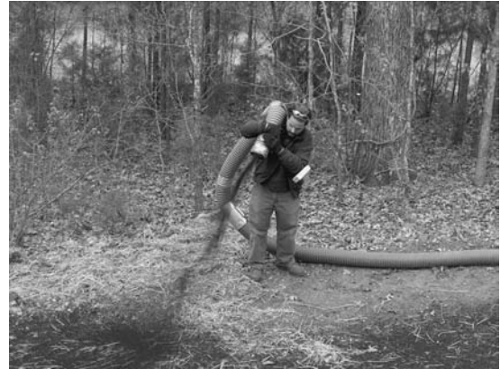
FIGURE 9. Application of compost mulch as a soil amendment and erosion control technique on disturbed soil.
