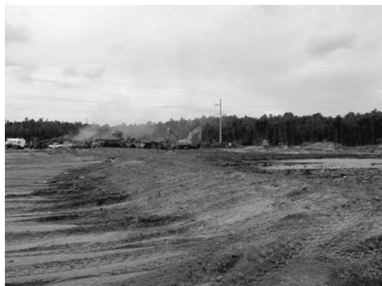
FIGURE 1. Clearing and mass-grading have become common practices that contribute to the degradation of natural processes on greenfield sites.
