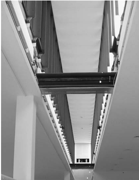
FIGURE 4. Skylight with constructive solar shading (gray) as constructed, seen from the floor and up into the skylight.
