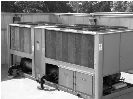
FIGURE 4. Packaged air source chilled water condensing unit located in a secured containment area.
