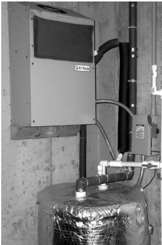
FIGURE 8. Air-source heat pump water heater connected to a standard hot water tank.
