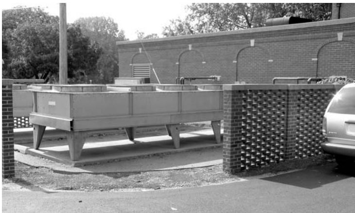
FIGURE 3. Air source condensing units located outside a building. Retaining walls are commonly required for security or noise control for larger systems.
