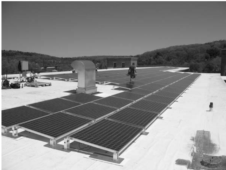
FIGURE 2. Flat roof low-slope PV mounting system.
