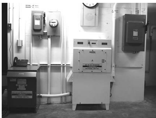
FIGURE 6. 30kW central inverter and BOS components.
