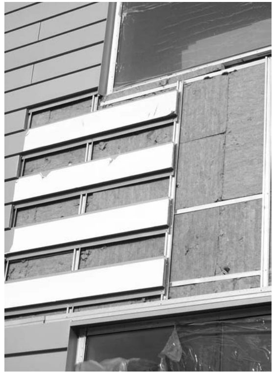
FIGURE 16. Zinc cladding panels on concrete wall backing with insulation in between (R-12 value). (Image: BCA/DSAI.)
