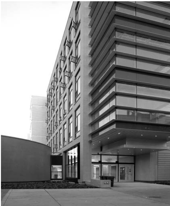
FIGURE 9. Windows on the North Façade are flushed with the exterior masonry wall to maximise daylight penetration. (Photo: Elizabeth Gyde, DSAI.)
