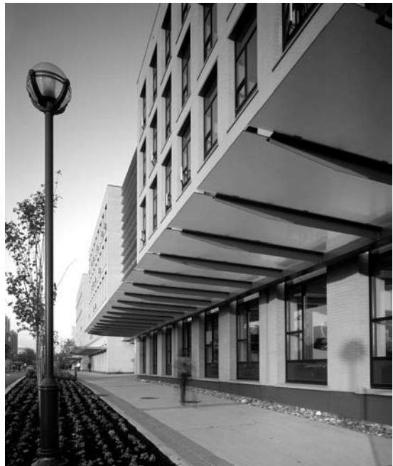
FIGURE 10. Windows on South Façade are recessed in the Masonry opening to provide shade. (Photo: Elizabeth Gyde, DSAI.)
