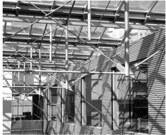
FIGURE 18. Savings in interior glazing and finishes of the atria offset the additional cost of the skylights. (Photo: Howard Waisman.)
