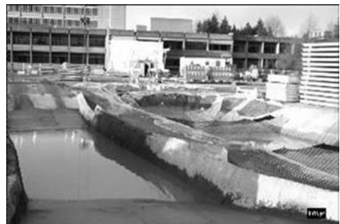
FIGURE 5. Temporary sediment basin and wheel wash. (Image: Aqua-Tex Scientific Consulting.)
