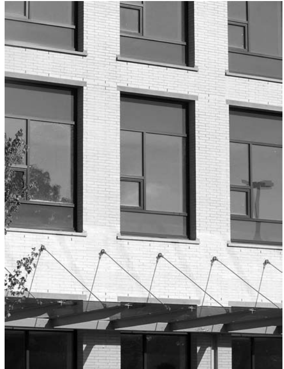
FIGURE 13. Brick veneer on north and south elevations. (Image: BCA/DSAI.)
