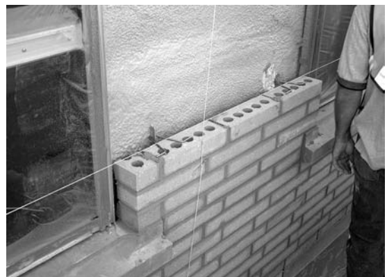
FIGURE 14. Brick veneer on concrete block wall backing with spray insulation within (R-12 value). (Image: BCA/DSAI.)
