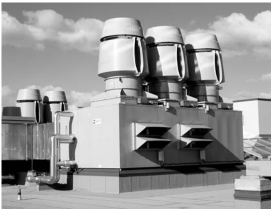
FIGURE 20. Strobic fans on the roof facilitate adequate dispersion of the exhaust by their high exit velocities. (Photo: Howard Waisman.)
