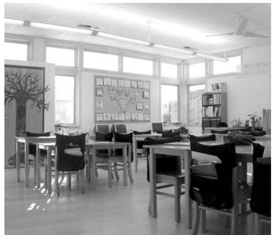
Continuous clerestory & view glass with direct/indirect fluorescent lighting.
