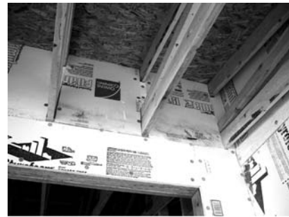
Insulation carefully inserted at trusses.
