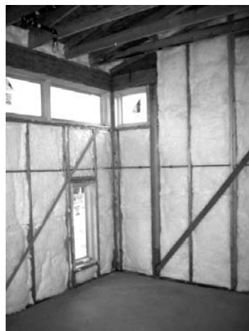
Exterior wall with building straps in lieu of sheathing.
