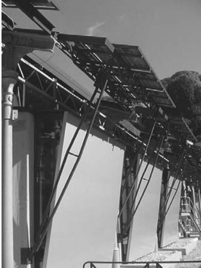
FIGURE 14. Photovoltaic canopies at the Children's Museum of Rome move to control shading on the south wall.
