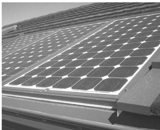
FIGURE 8. Photovoltaic laminates integrated into a residential roof with the aid of proprietary frames and showing a perforated metal batten to encourage air flow behind the modules. A corner of a solar thermal water heater is visible at left. (Source: PV Solar Tiles Pty. Ltd.)
