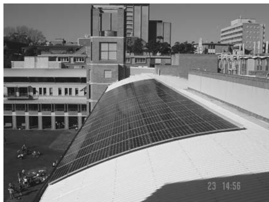
FIGURE 6. One of two sections of a 40 kW grid connected photovoltaic array mounted above the curved, corrugated metal roof of the “Quadrangle Building” at the University of New South Wales, Sydney. In this example, the photovoltaic modules were retrofitted and are not part of the building envelope. (UNSW Facilities Management 2006)
