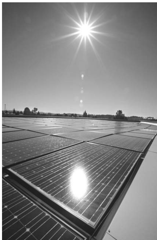
FIGURE 10. Interconnecting module system for flat roofs. (Source: PowerLight)
