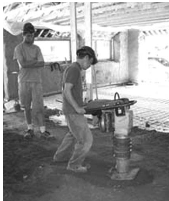
FIGURE 6. Laying and tamping earthen floor.
