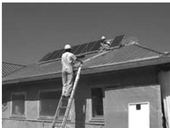
FIGURE 7. Installation of photovoltaic modules.
