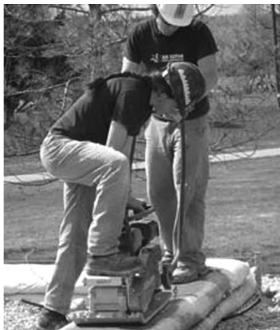
FIGURE 5. Placement and tamping of foundation.
