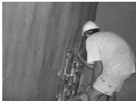
FIGURE 4. Pop bottle infill wall.
