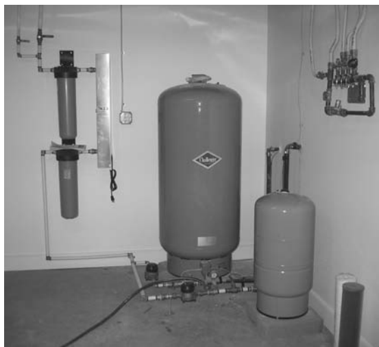
FIGURE 4. Water filtration equipment. Note two different storage tanks—one for rainwater and one for the backup system, which draws water from our well. The cylinders on the wall are the carbon filters; the long metal box next to the filters is the UV sterilizer.
