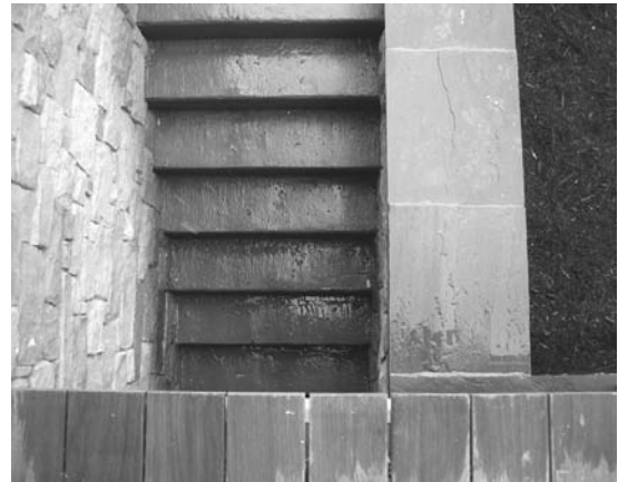
FIGURE 8. Reclaimed pavers and FSC certified cumaru decking.
