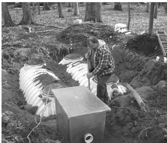
FIGURE 5. Installation of underground cisterns. The box in the foreground is the filtering roofwasher; the intake pipe at the bottom of the roofwasher will be connected directly to the downspouts.
