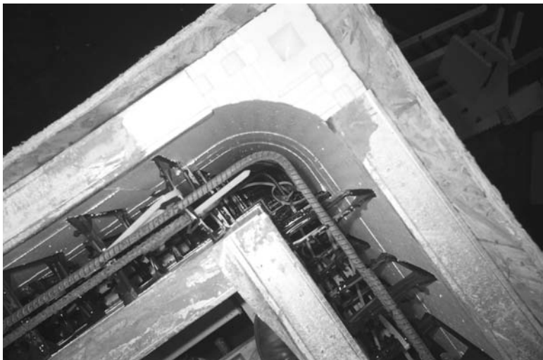
FIGURE 3. An outside corner ICF, top view. From outside (top of picture), materials are: OSB (screwed to fins that span through the ICF), expanded polystyrene foam, interior fins, steel rebar, and EPS foam.
